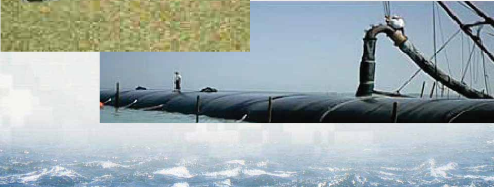
Geotube Filling Operation
