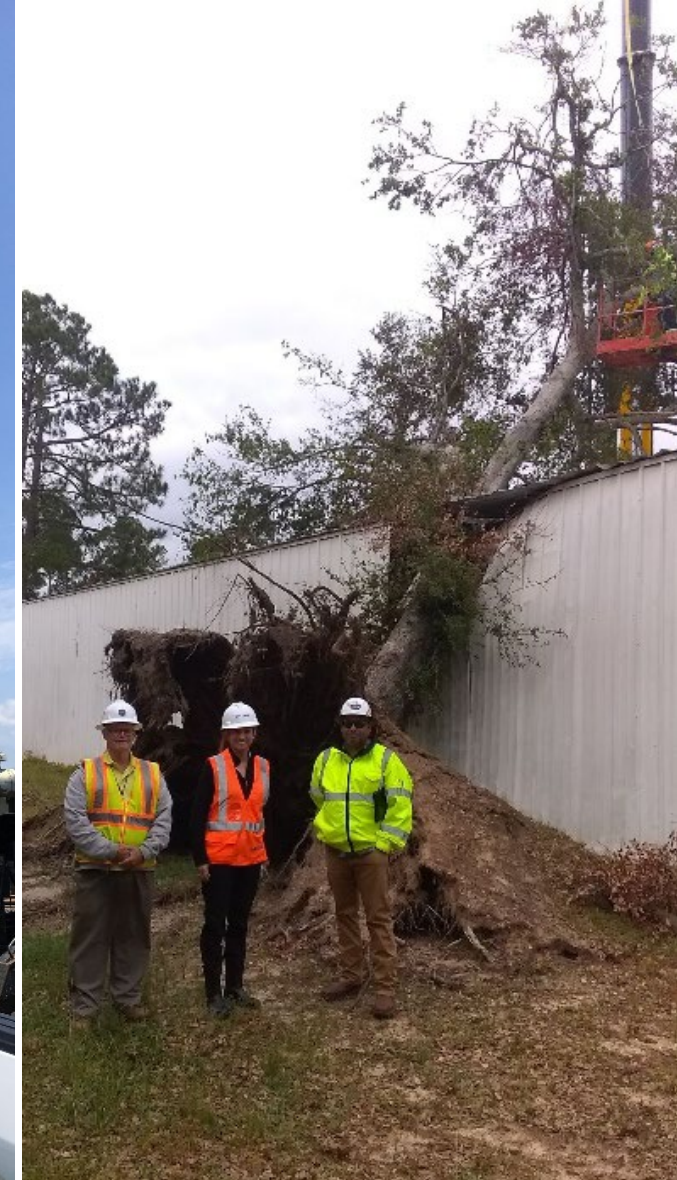
Hurricane Sally Recovery NAS Pensacola, FL
