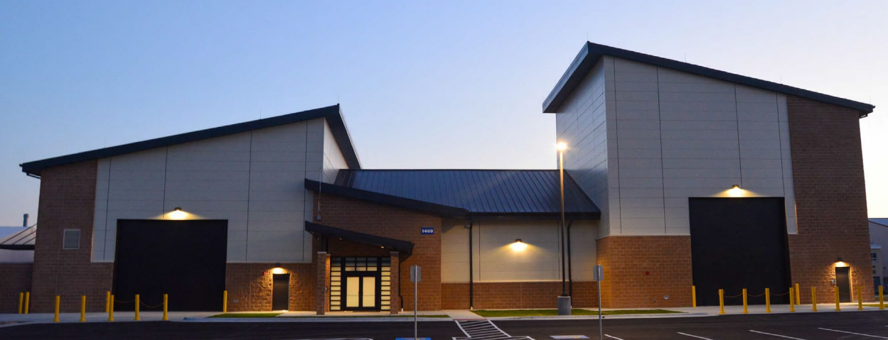
P-077 KC-130J Enlisted Aircrew Training System Facility NAS JRB Fort Worth, TX
