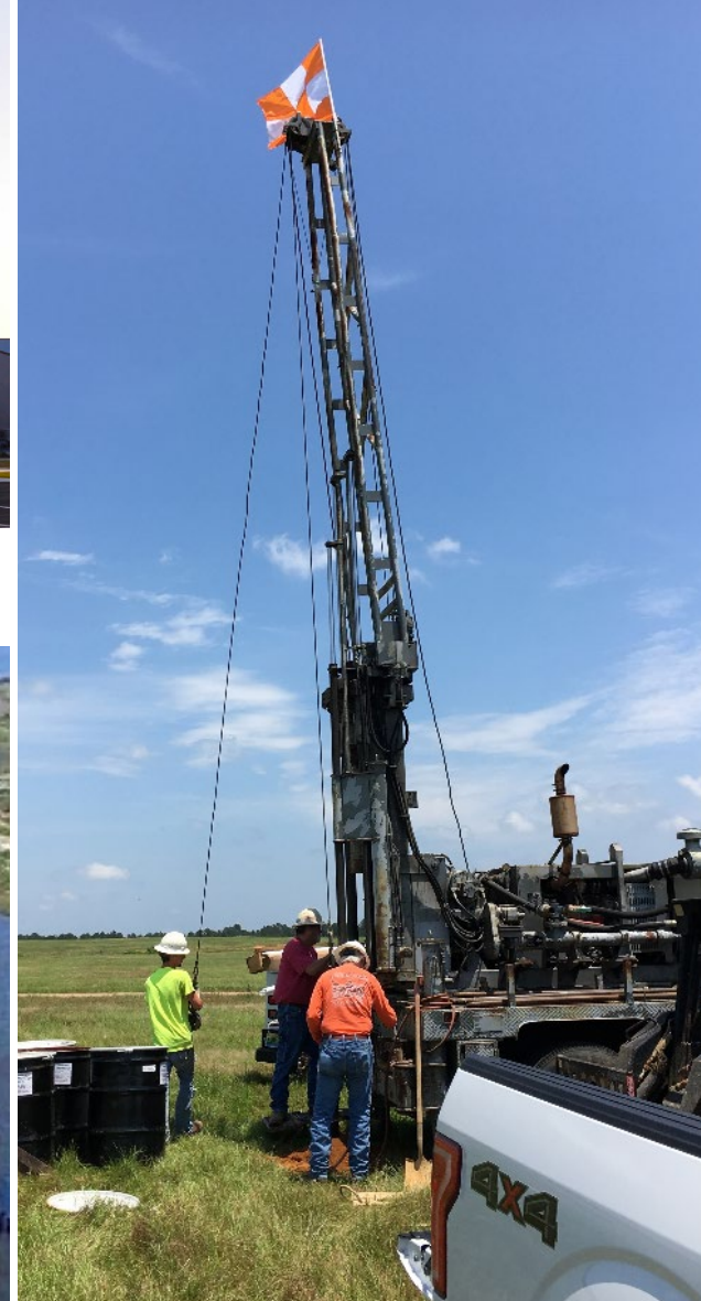
PFAS Site Investigation Well Installation, NAS Whiting Field, FL
