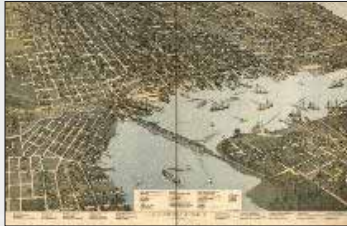
1884 | First permanent USACE office in Jacksonville (Captain W.T. Rossell)
