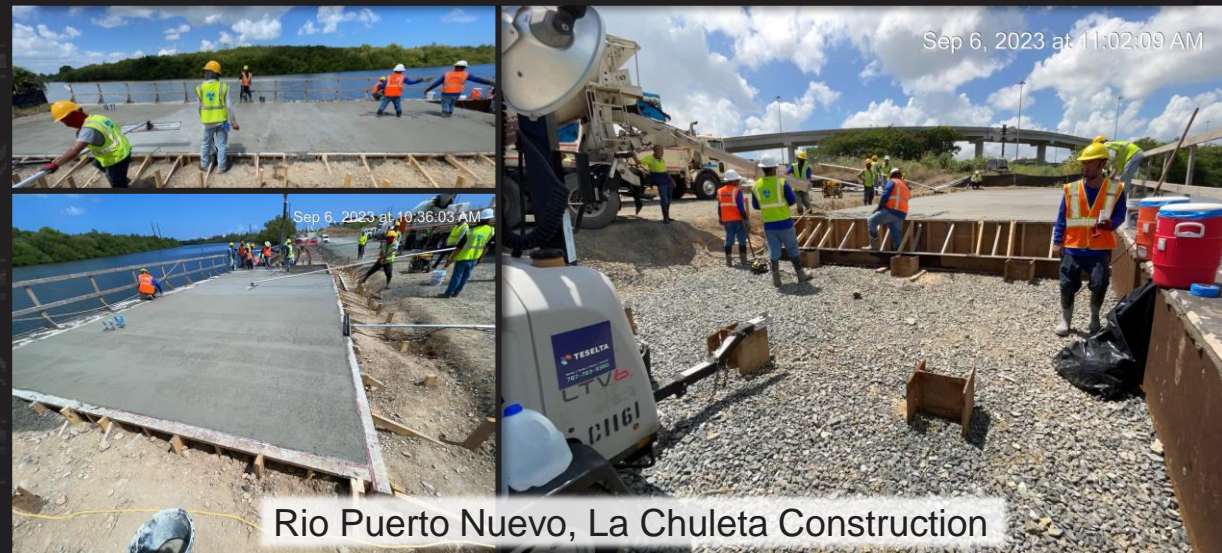
Rio de La Plata, Dorado Bridge and ACBM Toe Key Construction
